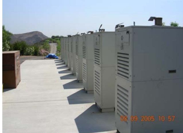
Figure 1. Calabasas Landfill - Microturbine Enclosures
