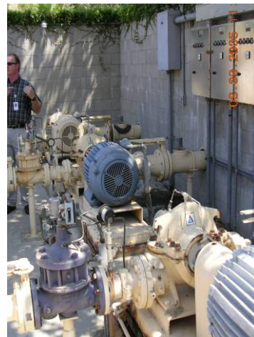
Figure 6. Irrigation Pumps
