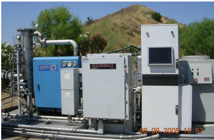
Figure 5. Gas Treatment Skid
