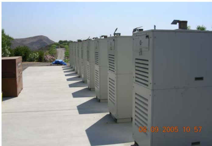
Figure 4. Microturbine Enclosures Alternative Energy Systems Consulting Inc.
