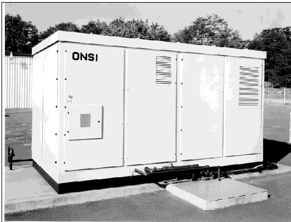
Figure 11 – ONSI 200 kW PC-25C Phosphoric Acid Fuel Cell Power Plant
