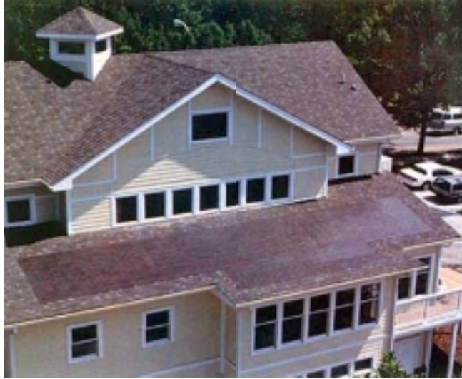
Figure 14 – Home with Uni-Solar Photovoltaic Shingles
