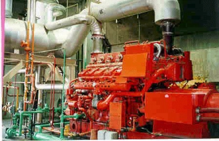
Figure 8 – 625 kW ICE Cogeneration Unit
