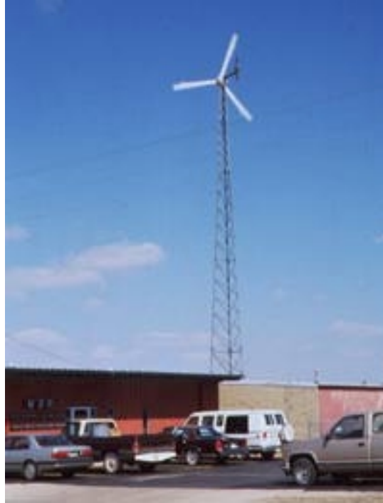
Figure 16 – 10 kW Bergey Wind Turbine
