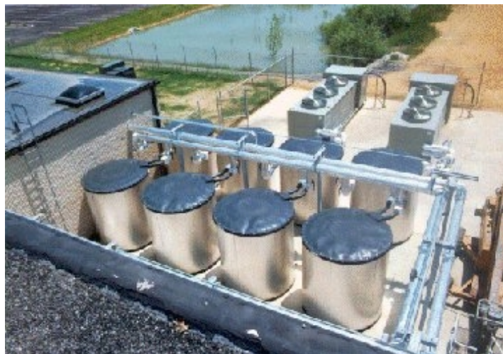
Figure 20 – Example Ice Storage System
